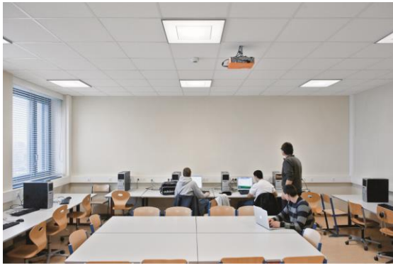
Image 3: The Höhere Technische Lehranstalt TGM Wien uses a flat LED ceiling luminaire with a bright ceiling aesthetic that acts like a natural skylight
